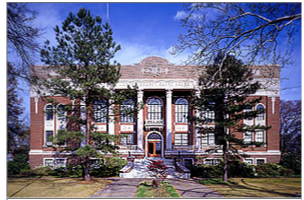
Historic Lonoke courthouse constructed in 1928.
